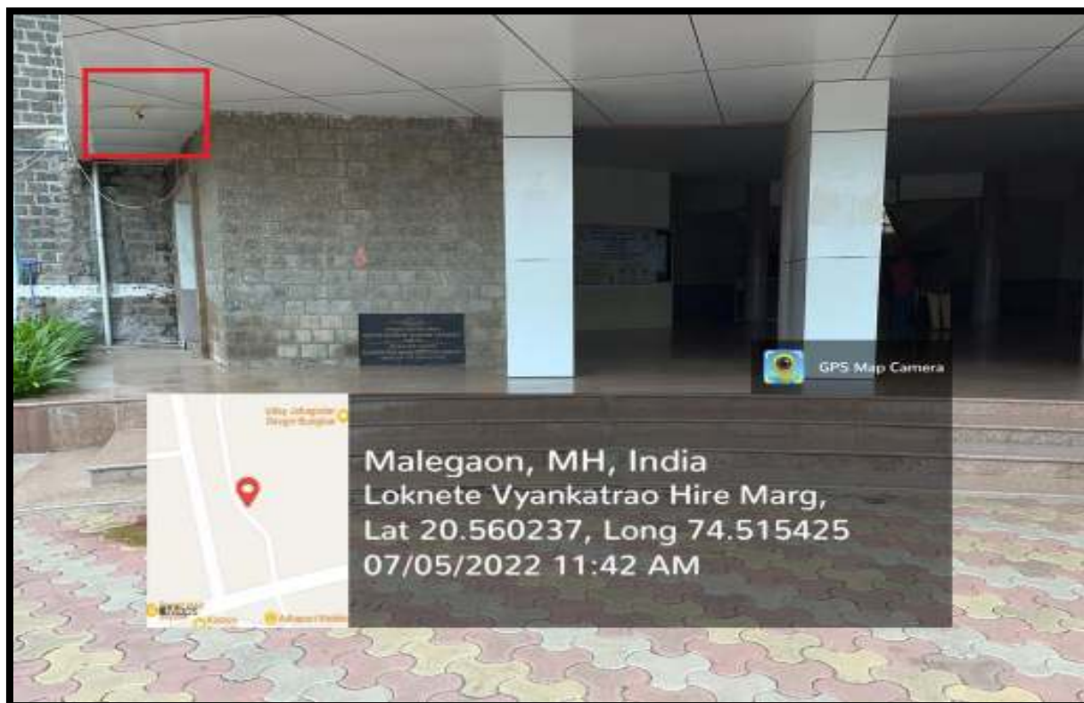
CCTV camera at main entry of college
