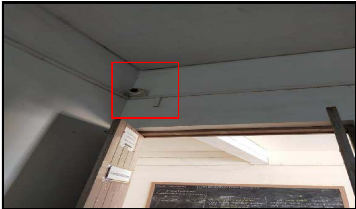
CCTV camera inside the Examination Department
